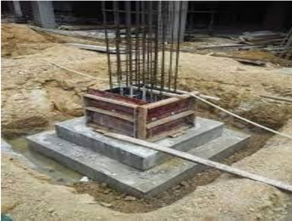
Figure 4 Stepped Footing for a Column
