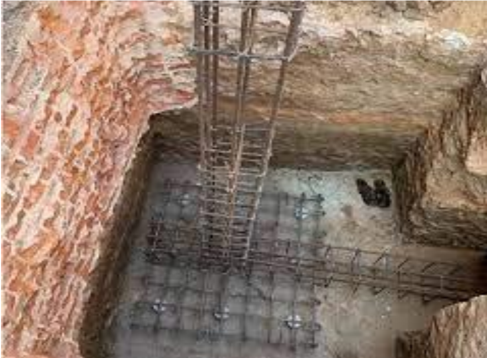
Figure 11 Cantilever or Strap Footing Image
