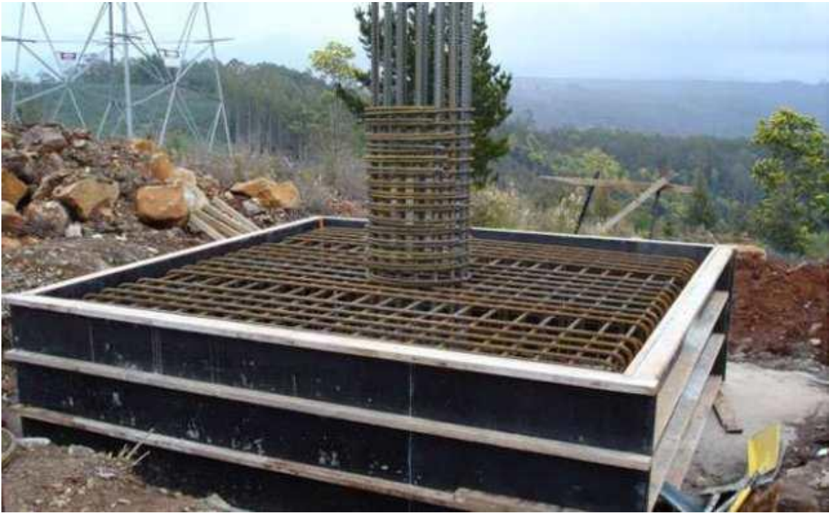
Figure 8 Grillage Foundation
